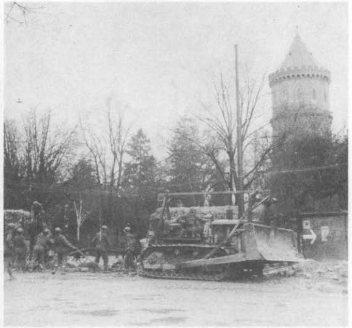
Engrs. tearing down longest road block in Calman, France, February 2, 1945
