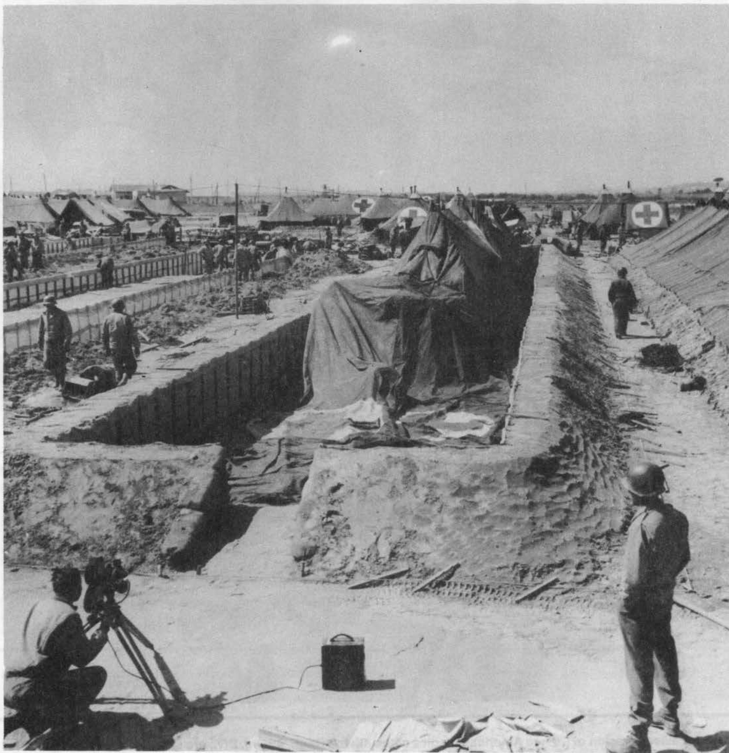
The 56th Evacuation Hospital shows a ward tent being erected. Note construction of side walls for tent. The digging in of Hospital Tents at Beachhead is necessary as German shell fire and bombing have hit American Hospitals several times. Fifth Army, Anzio Beachhead Area, Italy, April 2, 1944.
