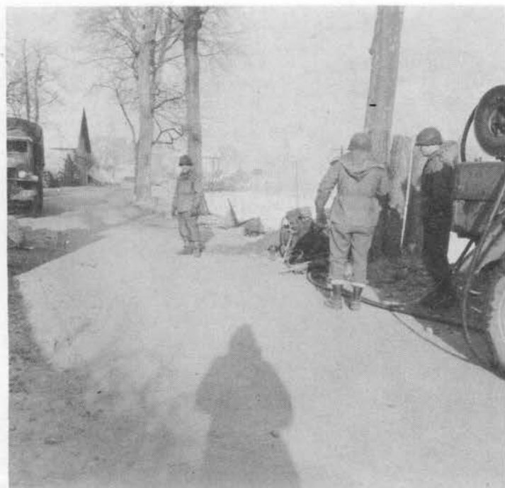
CO A, 10th Engr. BN constructing road block near Le Bonhomme, France, January 15, 1945
