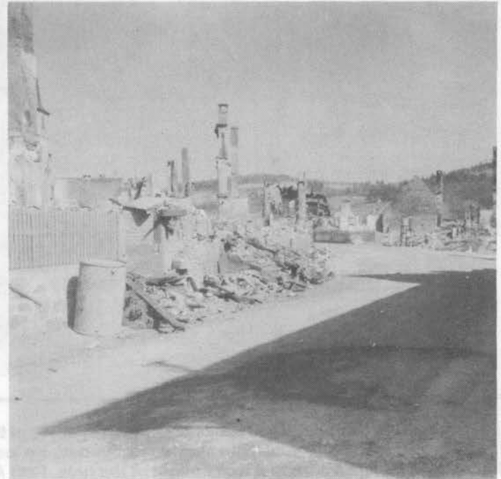
Wrecked building in Steinach, Germany, April 10, 1945
