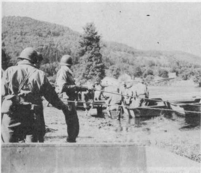
10th Engr. combat team constructs pontoon bridge near Remiremont, France, October 2, 1944
