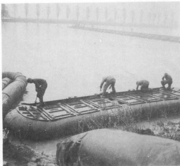
Men of the 2833 Engrs. and 163 Engrs. laying balk on a rubber pontoon before laying on the treadway. This rubber pontoon bridge was built between Worms and Bobenheim, Germany, March 26, 1945
