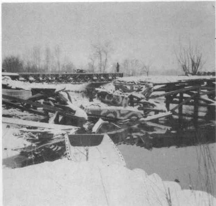
H-10 bridge between Ostheim and Riedwihr, France, collapsed under weight of Gen. Sherman tank, January 27, 1945
