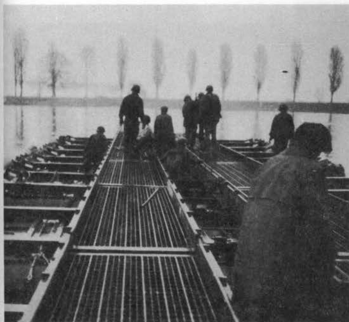
Men of the 2833 and 163 Engrs. are almost through with the treading bridge, shells and air bursts continue to come in between Bobenheim and Worms, Germany, March 26, 1945
