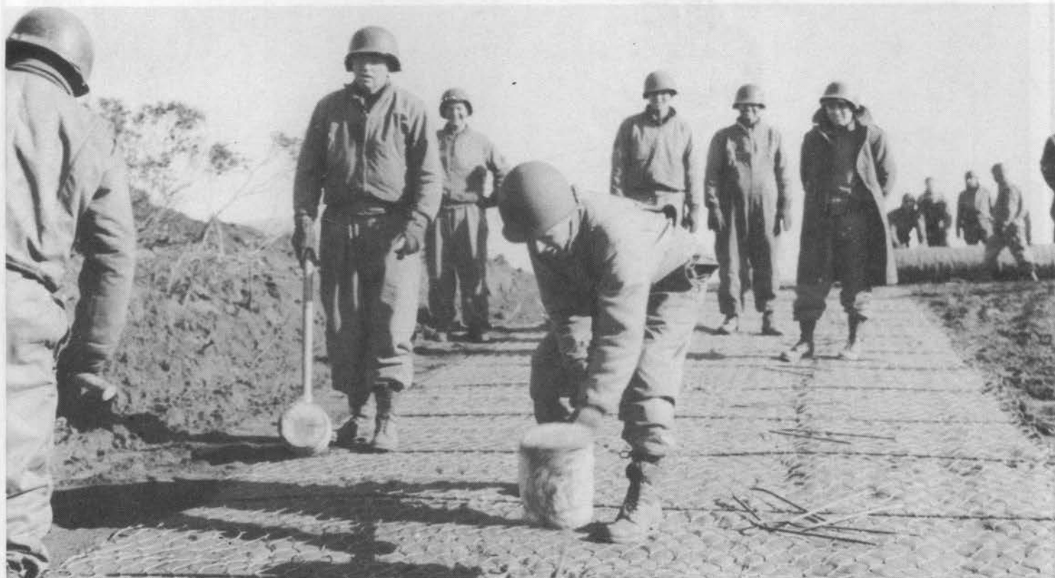
Part of the process of laying wire road mat, on the beach near Nettuno, Italy, is driving the stays into the sand to hold the mat firm. This is being done by men of an engineer regiment. February 6, 1944. Men of the 1st Bn., 540th Engr. Regt.
