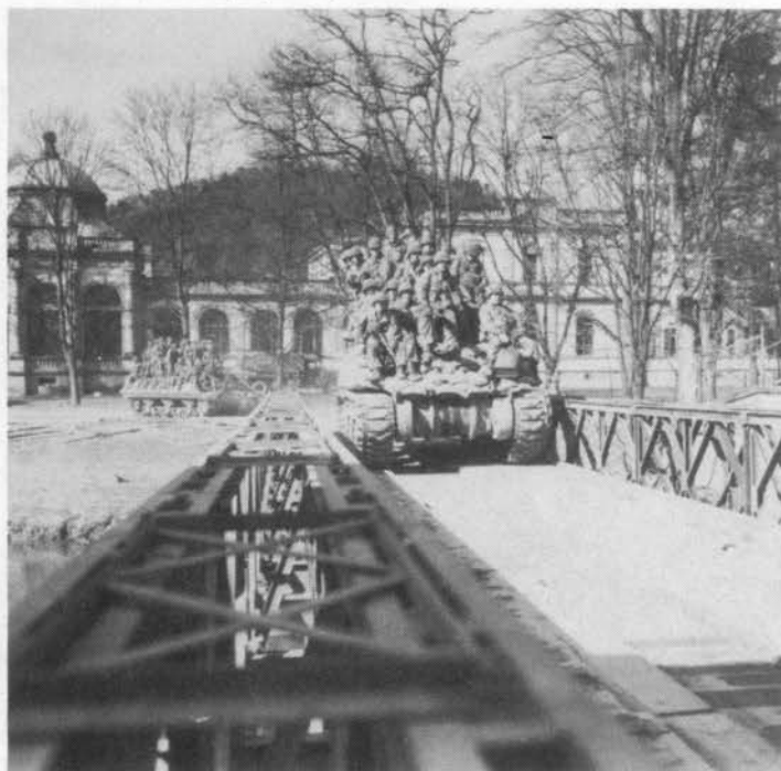
601st TP haul men of the 30th INF, 2nd BN across a Bailey bridge in the heart of Bad-Kissingen, Germany, April 8, 1945
