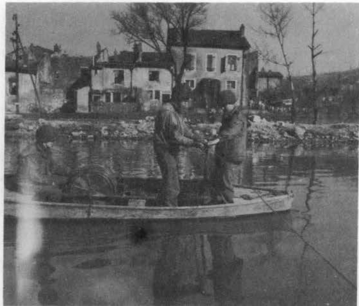
Stringing 12-pair cable across the Moselle River is this 3rd Signal Co. wire crew. Pvt. George W. Williams, T/Sgt. Earl H. Steiner and T/5 George W. Julian. Port a Mousson, France, February 24, 1945
