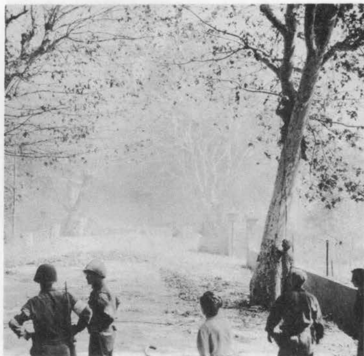
10th Engrs. construct by-pass outside Aix-En-Provence, France, August 20, 1944
