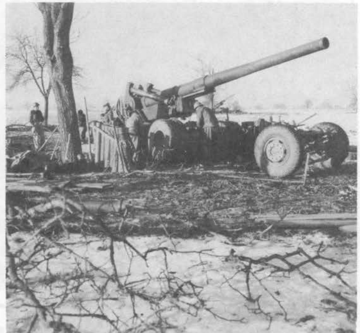
Digging in 155 long tour at Guemar, France, February 2, 1945
