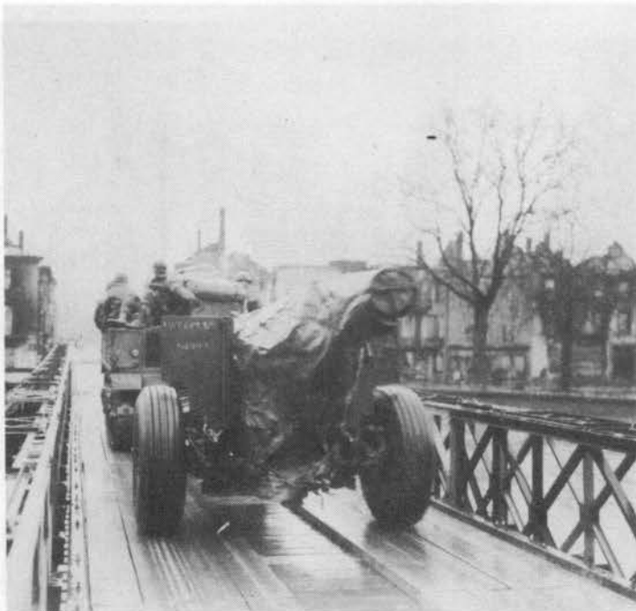
155 Howitzer passes over Bailey Bridge across Meurthe River, St. Die, France, November 23, 1944
