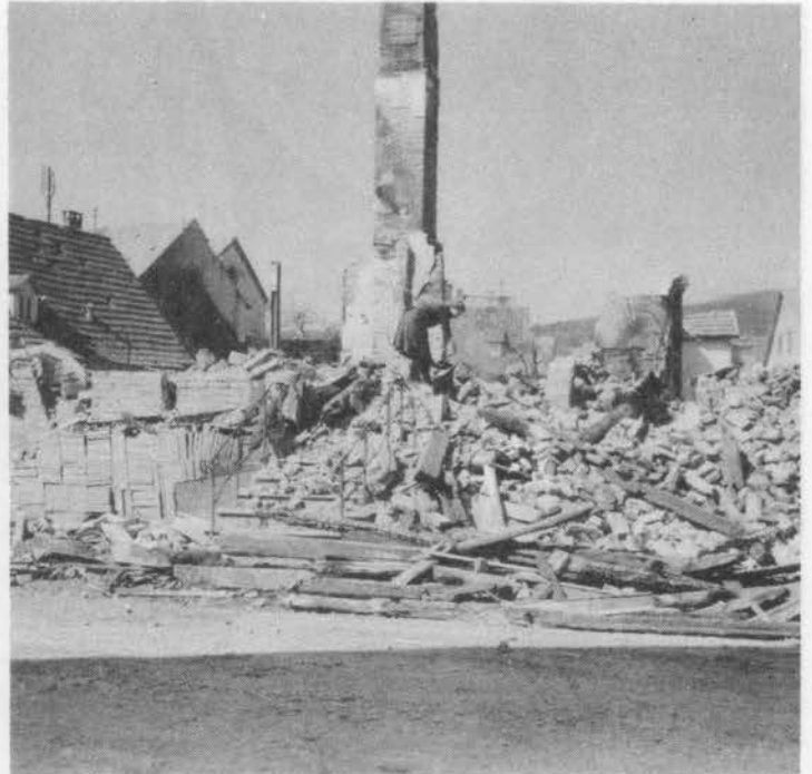
Civilians dig out wreckage of their home in Steinach, Germany, April 10, 1945
