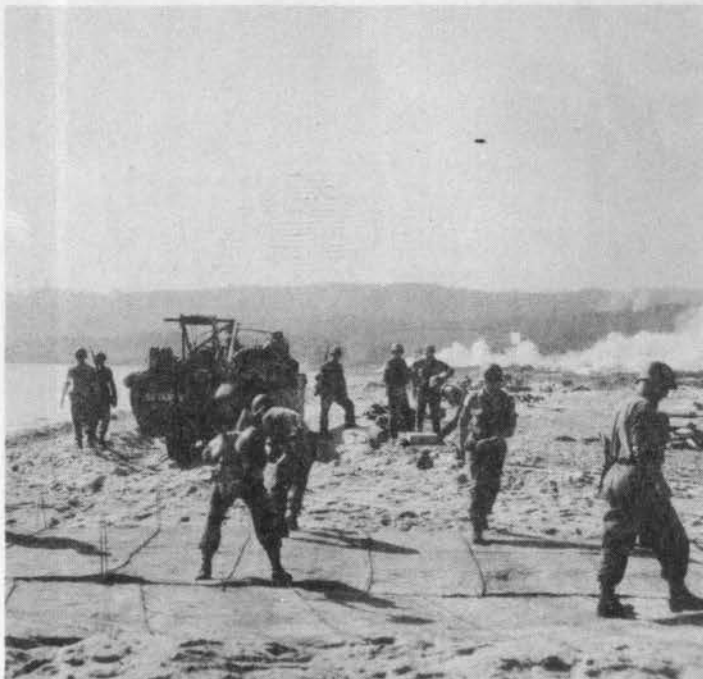
36th Engrs. constructing road on Yellow Beach, Southern France, August 15, 1944
