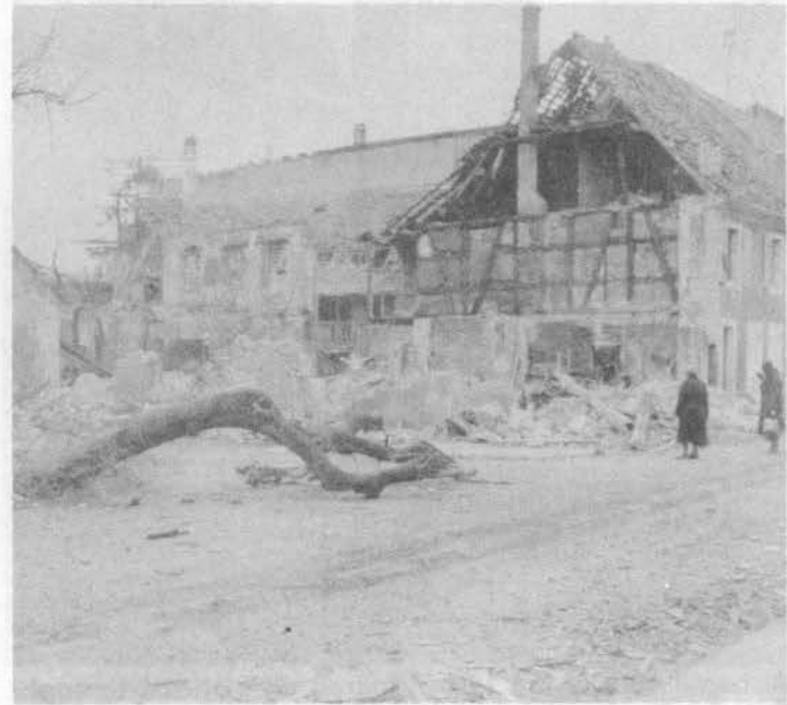
Bombed building in fortress city of Neuf-Brisach, France, February 11, 1945
